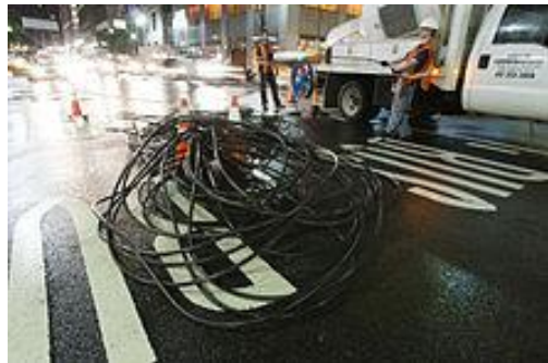
Stealth Fiber Crew installing a 432-count fiber cable underneath the streets of Midtown Manhattan, New York City
